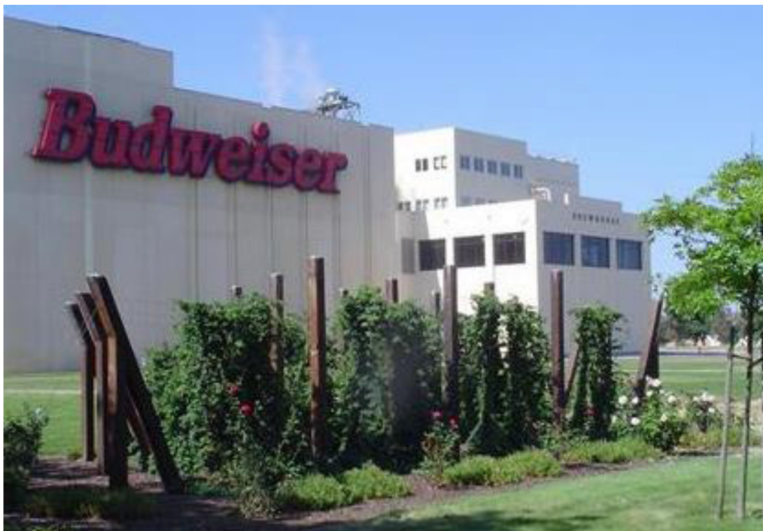
In 2008, the California Enterprise Development Authority issued $9.7 million in tax-exempt sewage facilities revenue bonds to Anheuser-Busch, producer of the popular Budweiser beers. This Budweiser Brewery in Fairfield, California, was upgraded thanks to tax-exempt bonds for sewage facilities. 118
