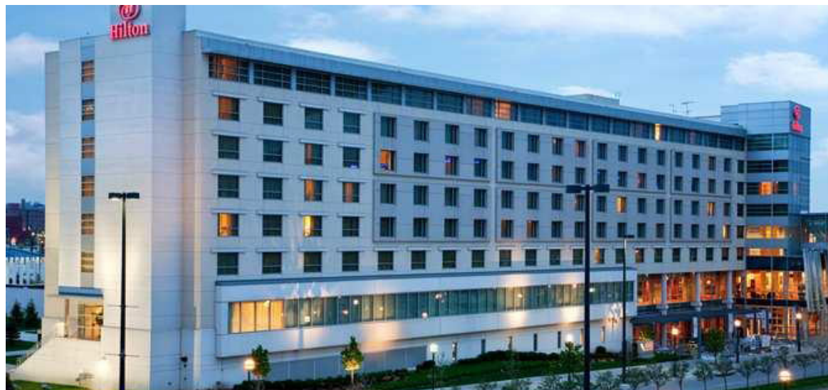
The 450-room Hilton hotel in Omaha, Nebraska received nearly $103 million in tax-exempt governmental bonds. 114
