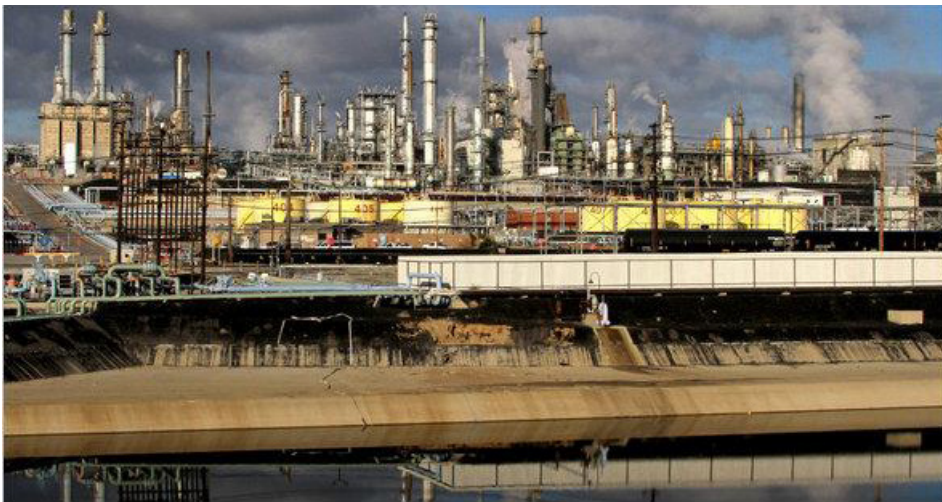
A ConocoPhillips refinery in Wilmington, California 5
