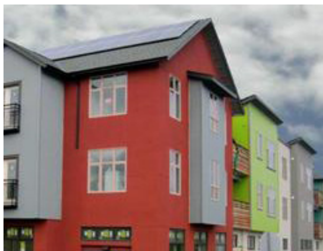
Plaza Point, an affordable senior citizen housing complex in California, built with both nearly $4 million in LIHTC and a $1 million USDA loan.
