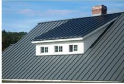
Figure 95-1: Building-Integrated Solar Energy System
